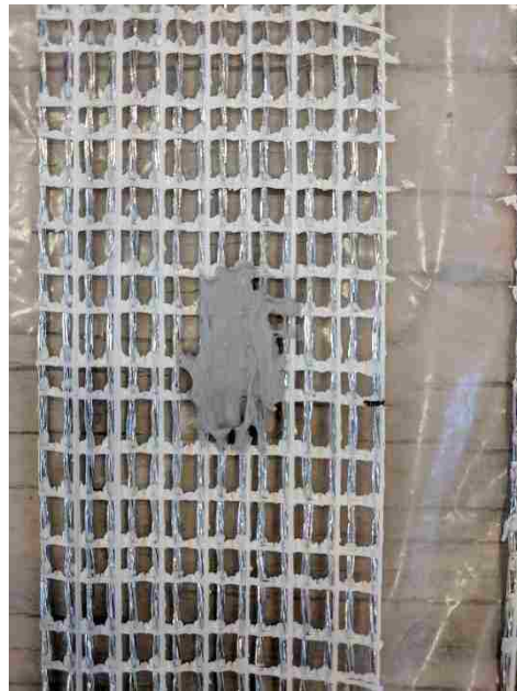
Figure 3.24. Hardened epoxy patch prior to sanding
