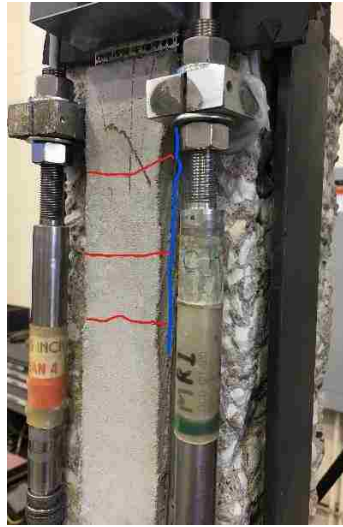
Figure 4.6. Longitudinal crack between internal and external matrix layer for specimen DS_330_50_C_1 (longitudinal crack shown in blue)
