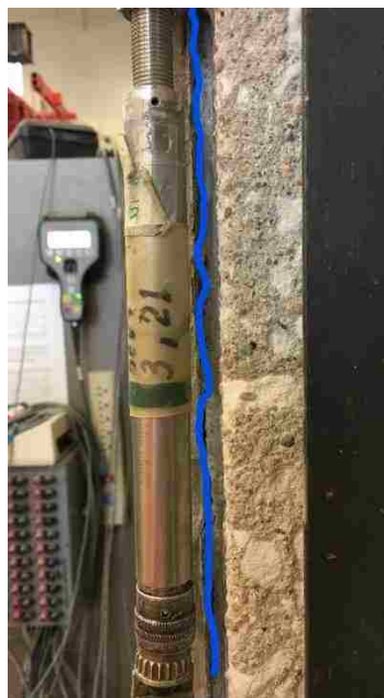
Figure 4.9. Side view of specimen DS_330_50_E_3 showing longitudinal crack between internal and external matrix layer (shown in blue)
